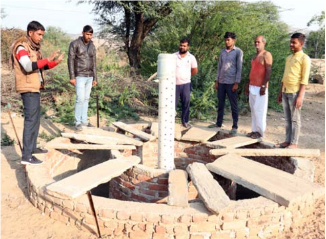
Community-based rainwater harvesting structures are constructed at common drainage line of the village catchment area found useful in increasing the groundwater table. A common water harvesting structure at village Ramsinghpura, Sikar.
